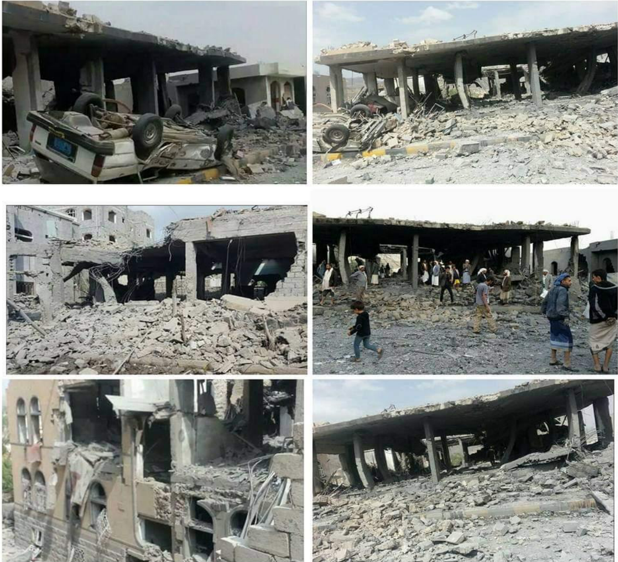
Figure1: Fare’s picture of the two targeted houses in Sana’a, 5 September 2015.
